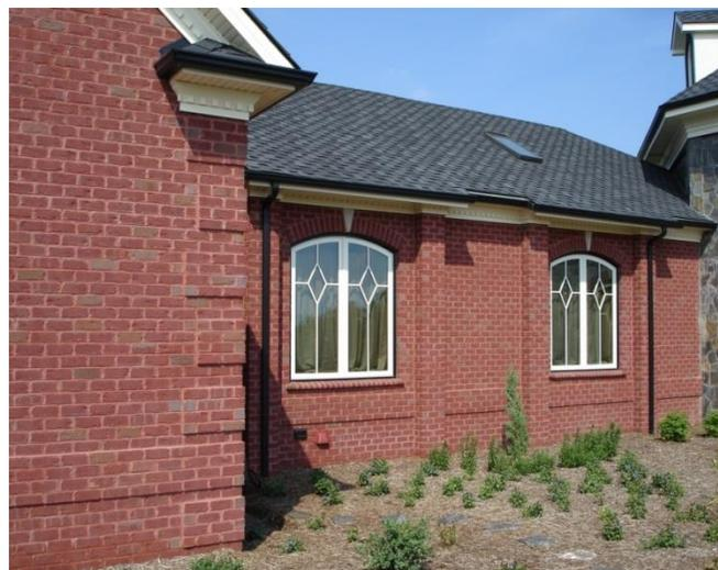
with molded brick products. Type N masonry cement mortars can be used when the specifier is experienced with a certain brand. Type S mortars should never be used with molded brick unless extraordinary circumstances require it.
